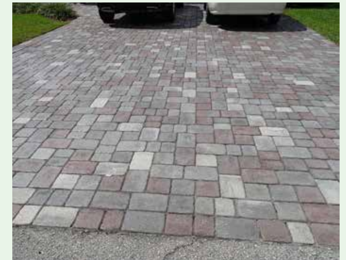
Adding permeable pavers to driveways is an attractive way to help reduce stormwater runoff.
