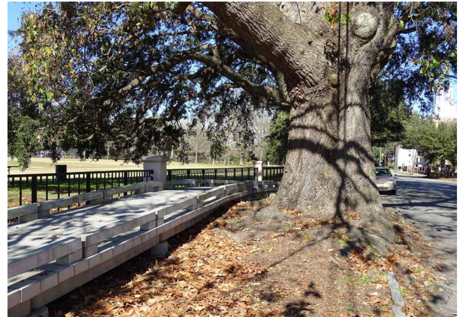
As this raised walkway shows, Charleston often makes significant efforts to allow large trees and sidewalks to co-exist.
