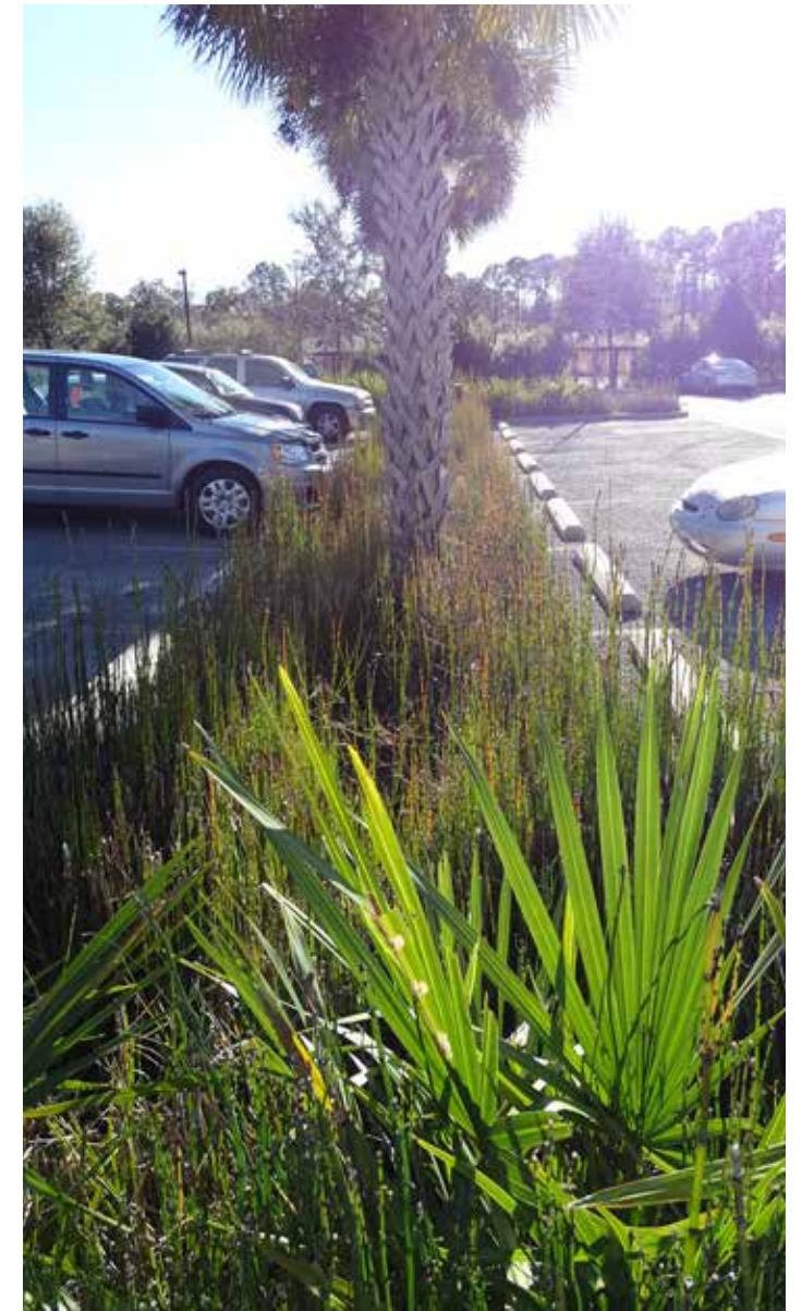
This parking lot in Charleston has both a permeable parking area and also a bioswale that captures and cleans the runoff.
