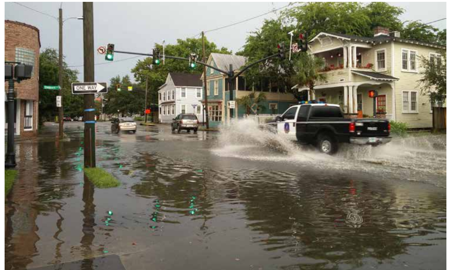
As this photo from August 2017 shows, even usual afternoon showers cause streets to flood.
