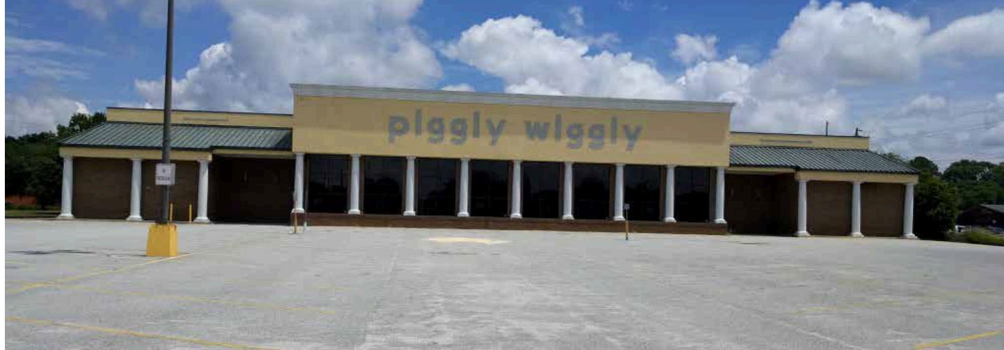
Excess impervious areas cause hot temperatures and runoff.
