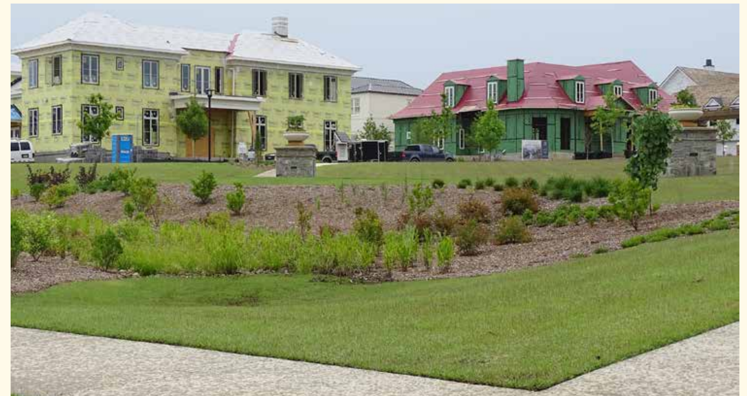
Bioswale in a new Greenville subdivision.
