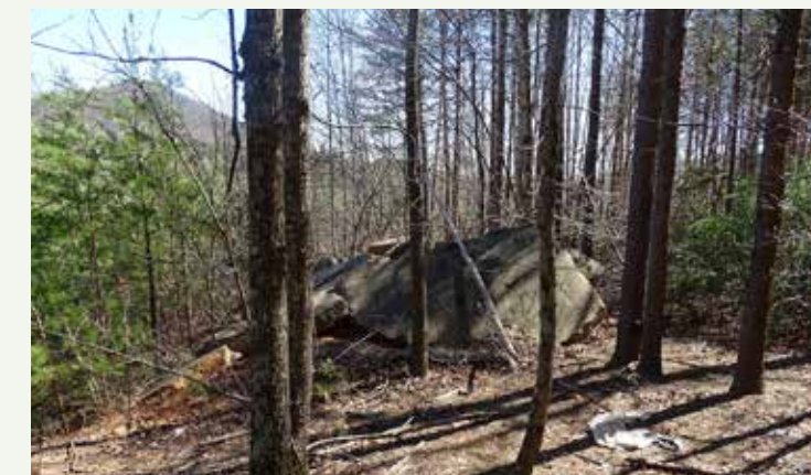
Ruins of a demolished structure with the mountain peak in the background.
