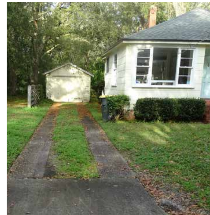
Residents can make a difference in runoff by limiting pavement as this residence has done with a partially green driveway.
