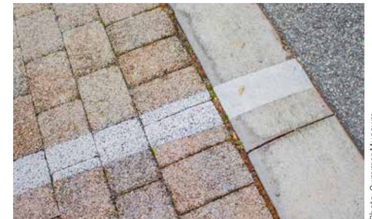
Permeable pavers in the Cummer Museum's parking lot allow water to infiltrate to the soil and reduce runoff while watering tree roots.
