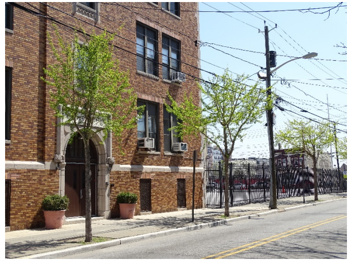
Newly planted Ginkgo trees that will become entangled in overhead wires as they grow.
